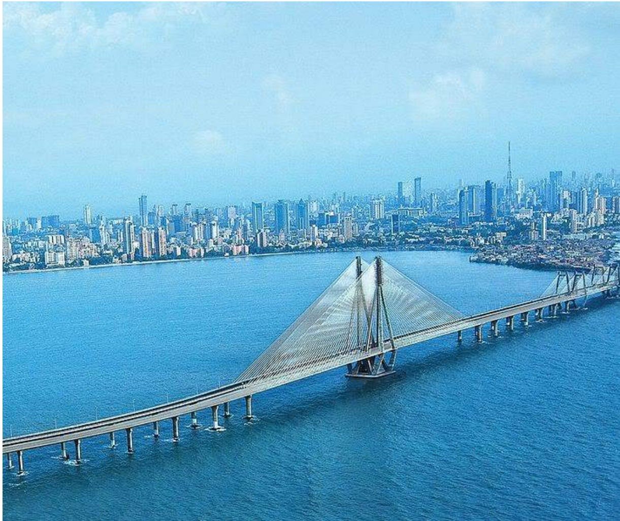
Snapshot of Bandra-Worli Sea Link Bridge (BWSL), Mumbai
