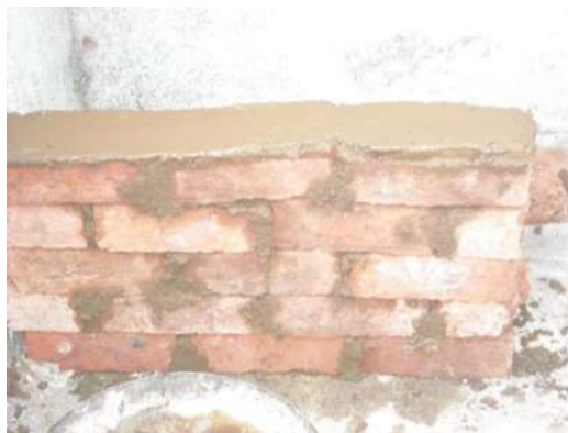
Fig 2. Side view of a section of cavity wall constructed
