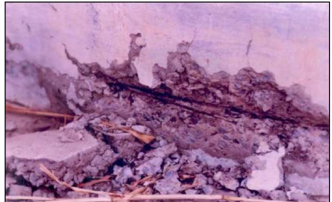
Fig. 13. Shaft at ground level
