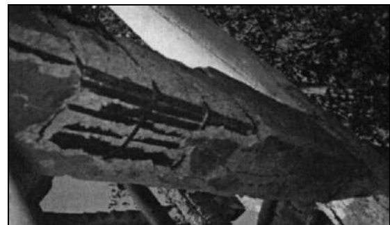
Fig. 9. Close-up of spalling of concrete in the bracing of one water tank
